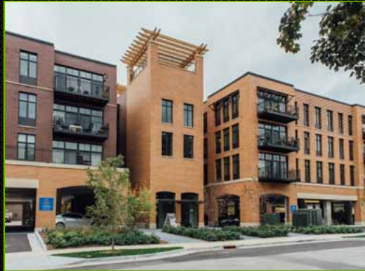
Beaumont Place Apartments
