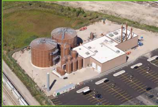
FCPC Renewable Generation Biodigester
