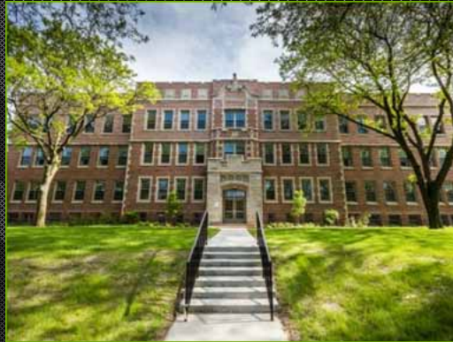
Bgemagen Building Renovation
