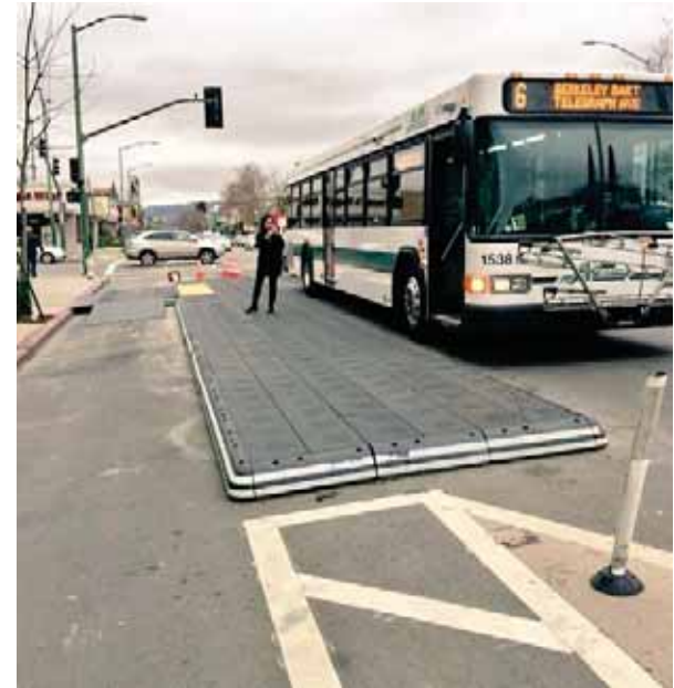
Snap-in-place plastic bus platform in Oakland, CA
